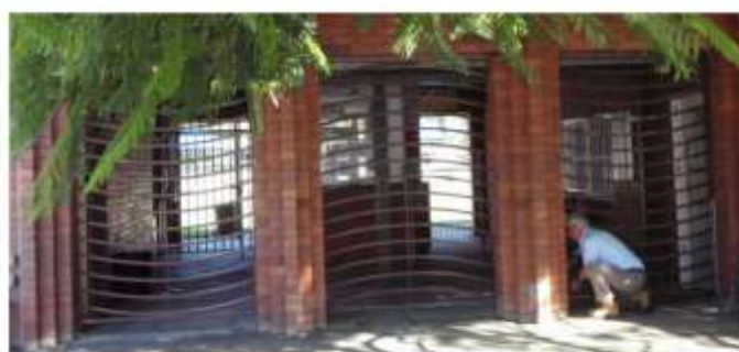
EXISTING METAL GATES- TO BE REMOVED
